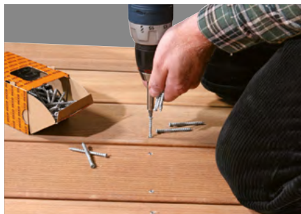
Fixing of decking
